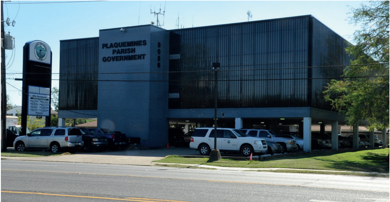
State asset inventories should include information on whether the assets have been mitigated or built to withstand hazard events. In this example, the Plaquemines Parish Government Building was constructed on pilings and includes storm panels that witheld winds up to 120 miles per hour. Image: FEMA
