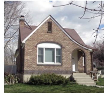
Salt Lake City home with braced chimney
