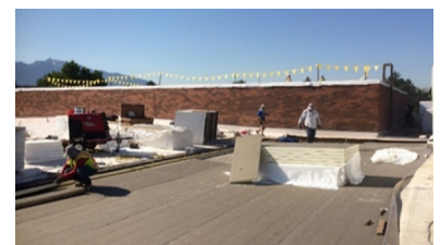
Murray School District Retrofit
